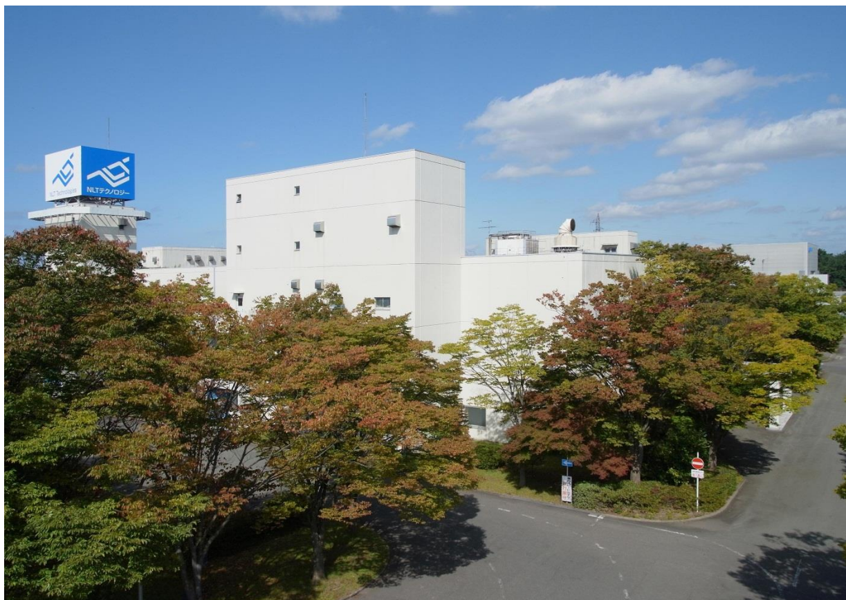
The Akita Plant
